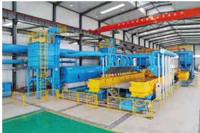
Lost foam production line equipment
