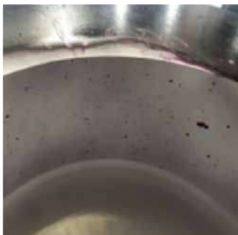
Fig 14a: Defective part excavated up to 135mm
